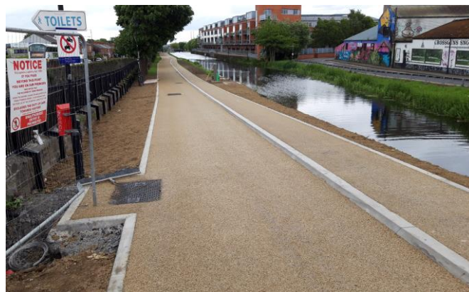
RCGP3: Final greenway surface near Cross Guns Bridge, Phibsborough
