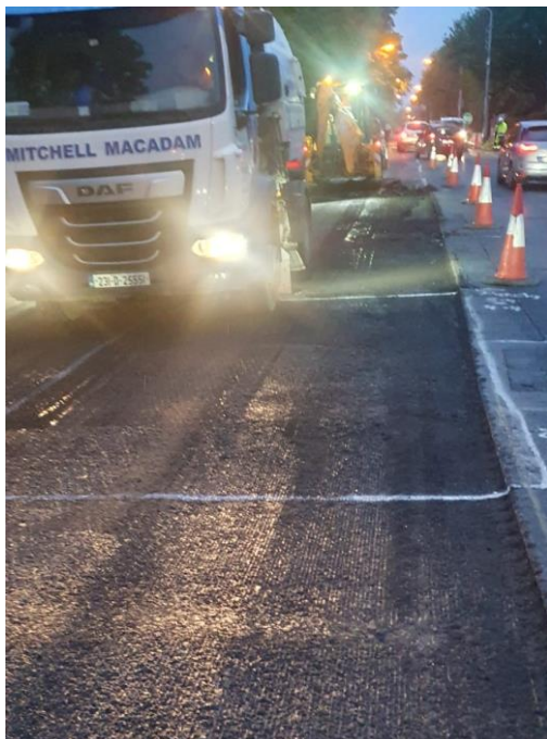
Road Maintenance Services resurfacing works on Nutley Lane
